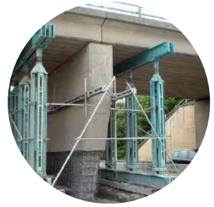
STRUCTURAL REPAIRS OF CIVIL STRUCTURES
