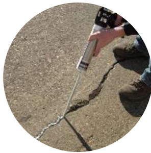
PU & ACRYLIC BASED CRACK FILLING
