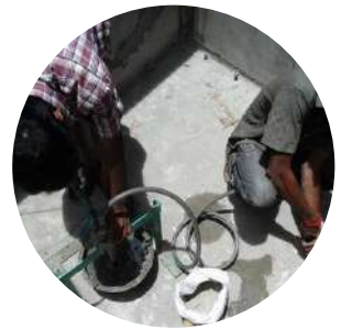
INJECTION GROUTING - PU & CEMENTITIOUS
