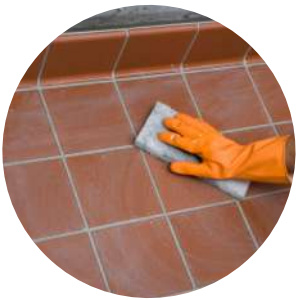
EPOXY GROUT - TILE JOINT FILLING
