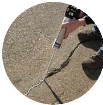
PU & ACRYLIC BASED CRACK FILLING
