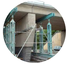
STRUCTURAL REPAIRS OF CIVIL STRUCTURES
