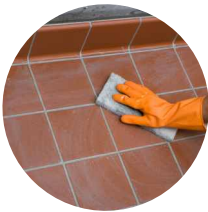
EPOXY GROUT - TILE JOINT FILLING
