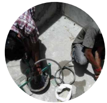
INJECTION GROUTING - PU & CEMENTITIOUS
