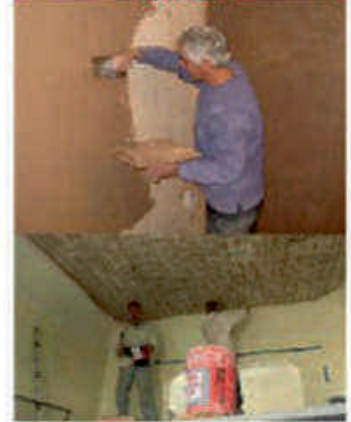
Wall Plastering Interior Exterior
