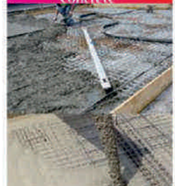
Reinforced Cement Concrete
