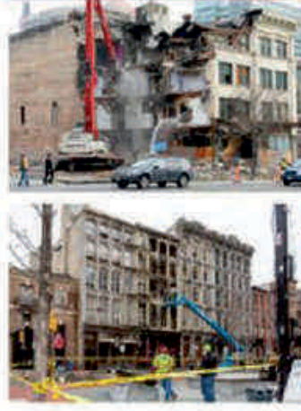
Old Building Demolishing
