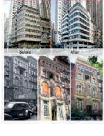
New Building Renovation
