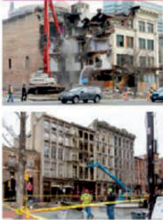
Old Building Demolishing
