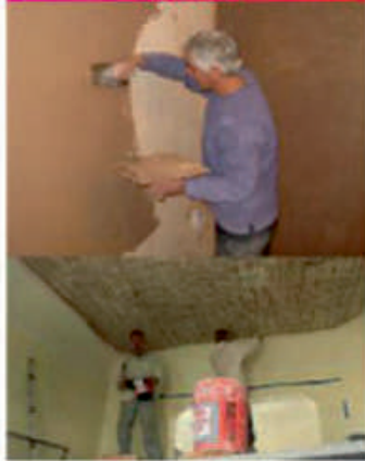
Wall Plastering Interior Exterior
