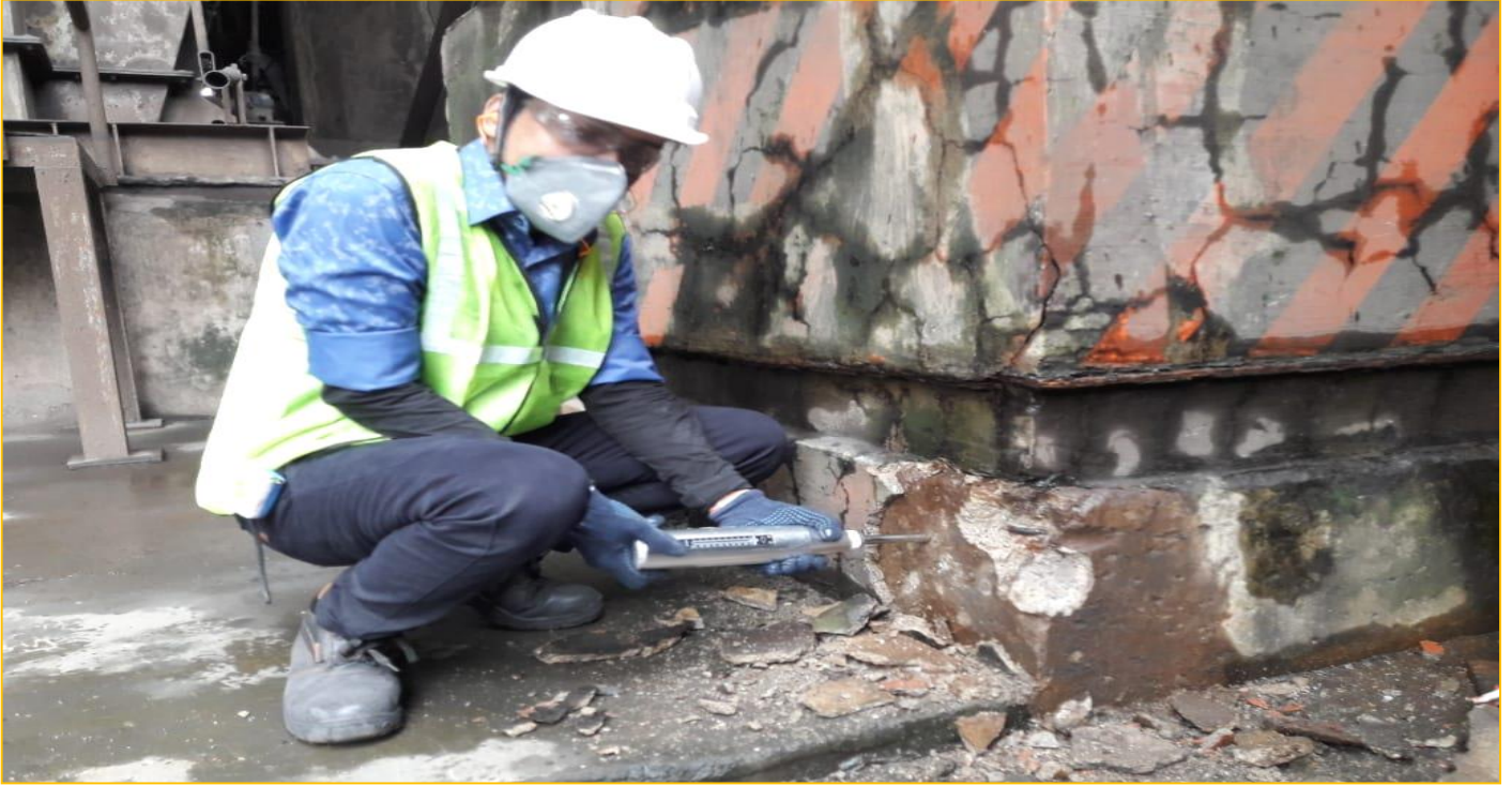
REBOUND HAMMER TEST
